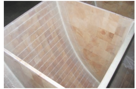
The Kerfs on the inside of the bridgedeck panel.
