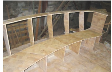
Aft cockpit seat being assembled.
